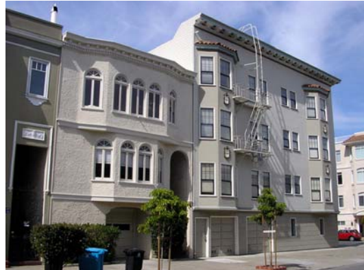
(b) Example of closely spaced buildings.
