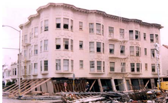
(f) Loma Prieta building damage.
