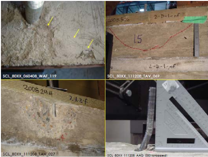
Image 2 – Concrete side break-out development.
