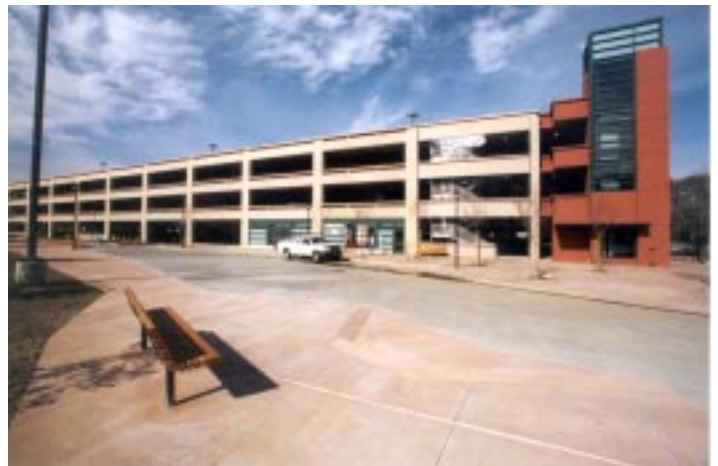
Stanford Shopping Center: Parking Structure
