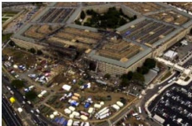
beginning in September 1941. The five-story building is a cast-in-place concrete space frame. The Boeing 757 airplane entered the first story, and the debris traveled approximately 300 feet through the structure. Although a portion of the exterior ring did collapse within a half-hour of the impact, the structure exhibited remarkable toughness.
