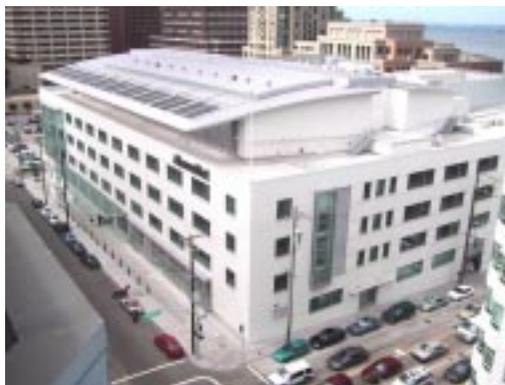
The project presents an example in the application of seismic isolation technology to transform a 1940's non-ductile reinforced concrete warehouse and its conversion into a state-of-the-art Internet "co-location" facility with the goal of continued operation following a major earthquake. The completed Internet Service
