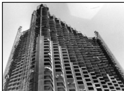
Bank of America Building, 555 California, during construction in 1968 (courtesy of EERI)
